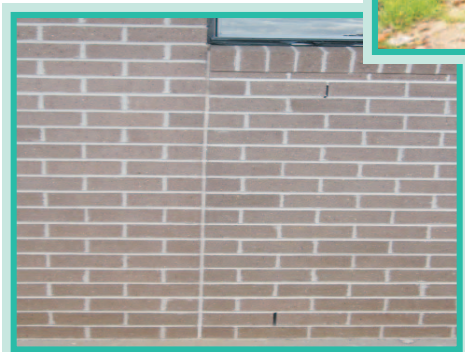
External Joint Sealing on Houses
