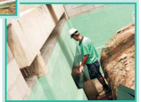
Commercial Retaining Wall with Below Ground Waterproofing
