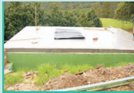
Residential Retaining Wall
